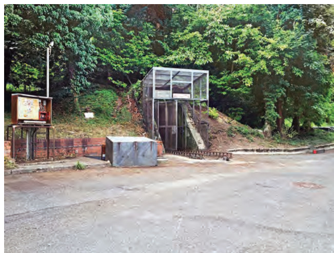
The emergency exit and equipment winch. The rails for the equipment trolley are seen. Photo Rob Jacobs
